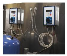
Dual peristaltic pump assembly, RC-0021-0002
